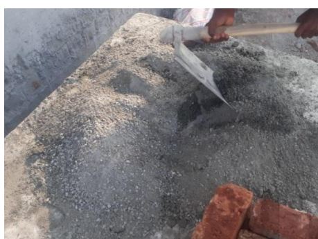
Fig.3. Dry mix of soil ,cement and coarse aggregate
